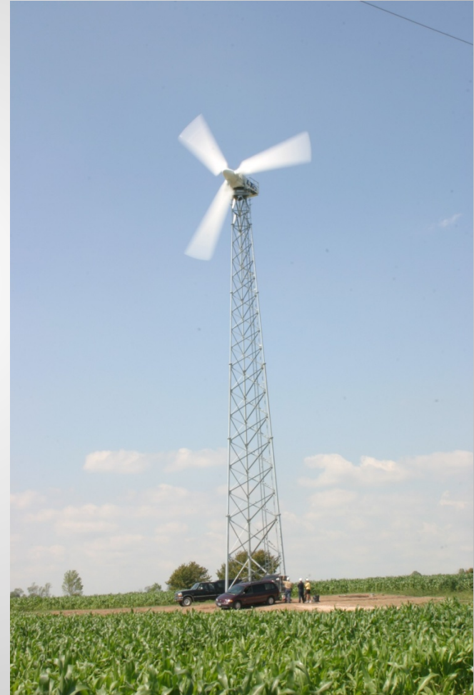
65 kW Vestas V-15 at Lakeshore Technical College, Manitowoc Co.
